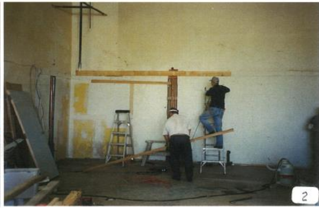
The first board installed during construction
