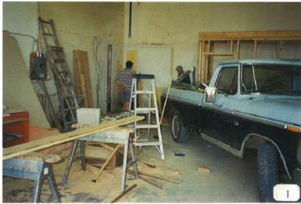
The area gets gutted
